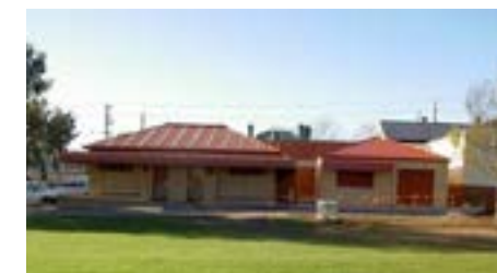
Kiosk completion in June 2007
