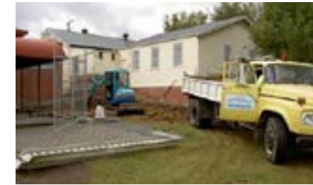
Footings for Kiosk started in Feb 2006
